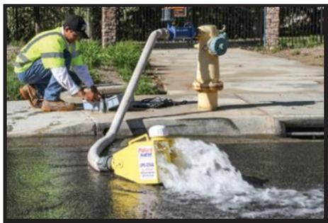
Flushing the water mains improves water quality by removing sediment that slowly builds up at the bottom of the water main over time.
